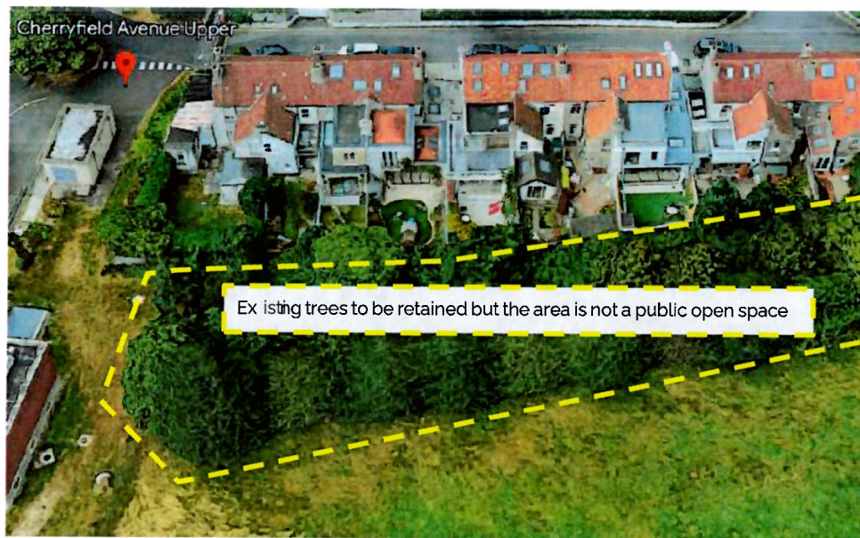
Fig.53: Client's residents most impacted by Block D
